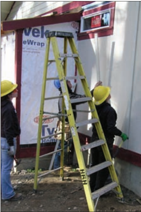
Thursday crew members work on siding Darlene Keefe photo
